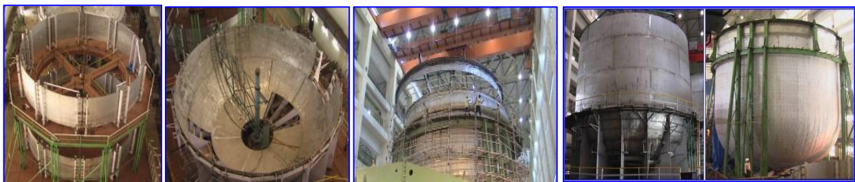
Figure-3: Main Vessel and Safety Vessel of PFBR fabricated at Kalpakkam site
