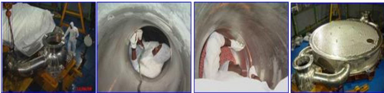
Figure-5: Welding of Grid Plate to Primary Pipe
